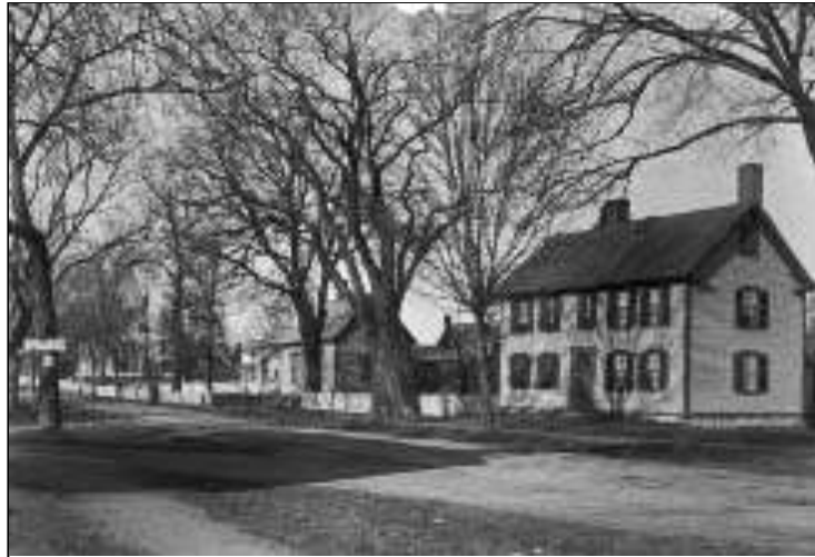
Main Street looking south: Larch Row sign at left, Ben Young, George Alley and Elbridge Kimball houses ( right to left ), 1891. Photo courtesy Wenham Museum
