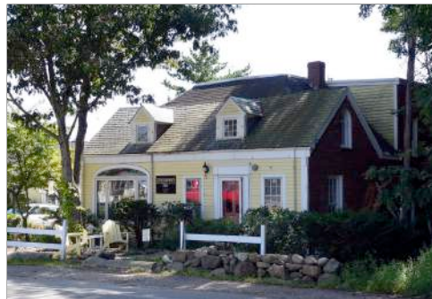
Bay window is where the Jenny station garage door had been. Photo J. Hauck, 2011.
