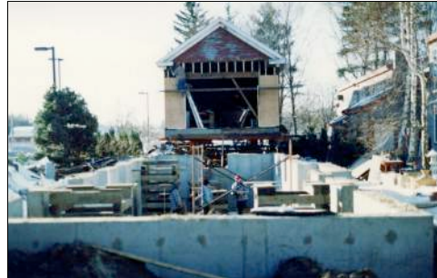
Placing shed on basement foundation, 1990. Photo D. Costin
