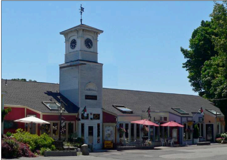
At street level, there are five shops. On second floor, there are four more businesses. Photo J. Hauck, 2012
