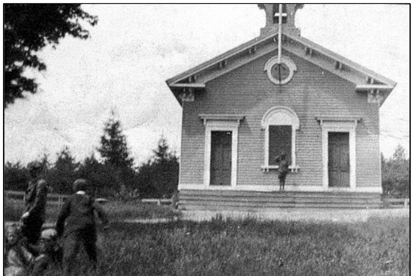
South School , also called Center School, was on Main Street, between what now are 454 and 484 Bay Rd. Photo, Hamilton Historical Society.
