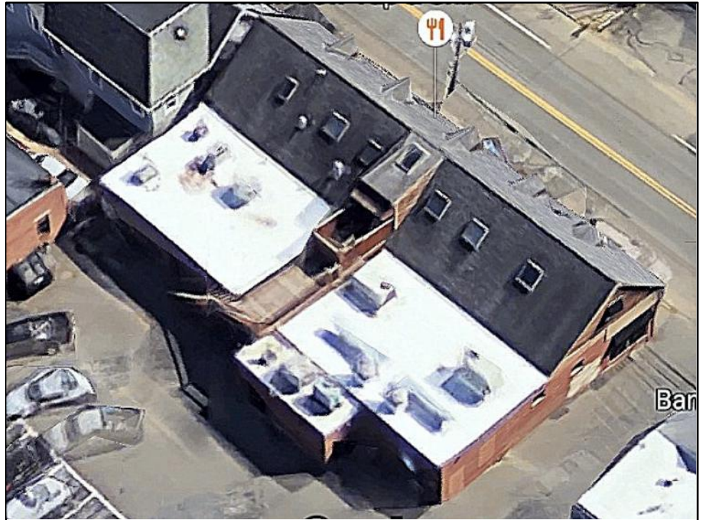
A second floor was added , in 1994, to provide more rentable space. Extensions behind the street side stores provided more space. Exterior stairs, built at the back, became a second egress for offices. Photo, Google, 2015
