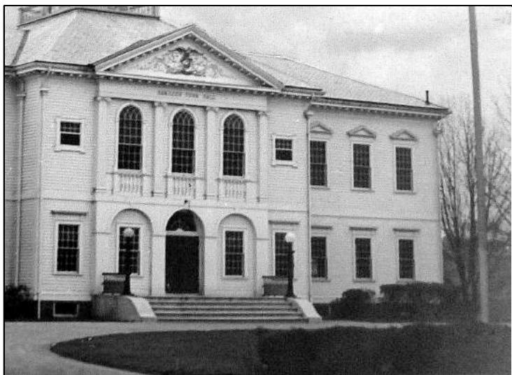
1897 -- Constables had an office to the right of entrance to new Hamilton town hall. Photo, Hamilton Historical Society.
