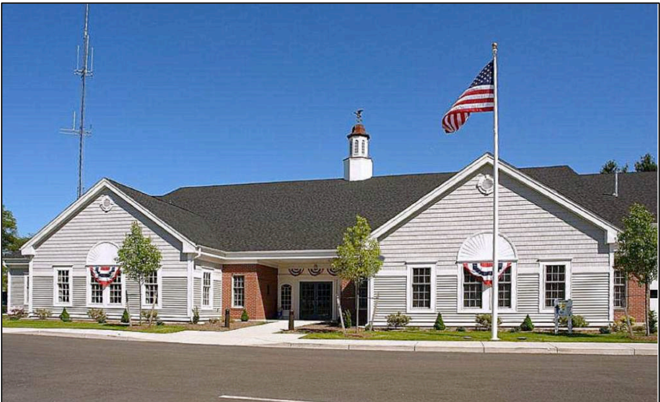
Hamilton Police Department occupies the left section of the Hamilton Emergency Center, built in 2008. Fire Department is in right section and garage to far right ( not shown ). Photo, Hamilton Emergency Center, 2014
