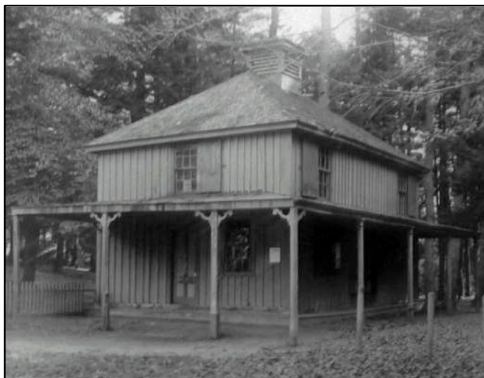
Asbury Grove police station, built in the late 19th century, no longer remains. It was a small, two-story building opposite the dining hall. There now is a garden on the site of the old station. 55 As the number of visitors decreased in the 20th century, there was no longer a need for police supervision. By the 1940s the Grove's superintendent and other residents were granted the status, from the Hamilton Police Department, to be "special police." This gave them legal control over any wrongdoing. 5 The Hamilton Police Department now has responsibility for the Grove. Photo, Hamilton Historical Society.
