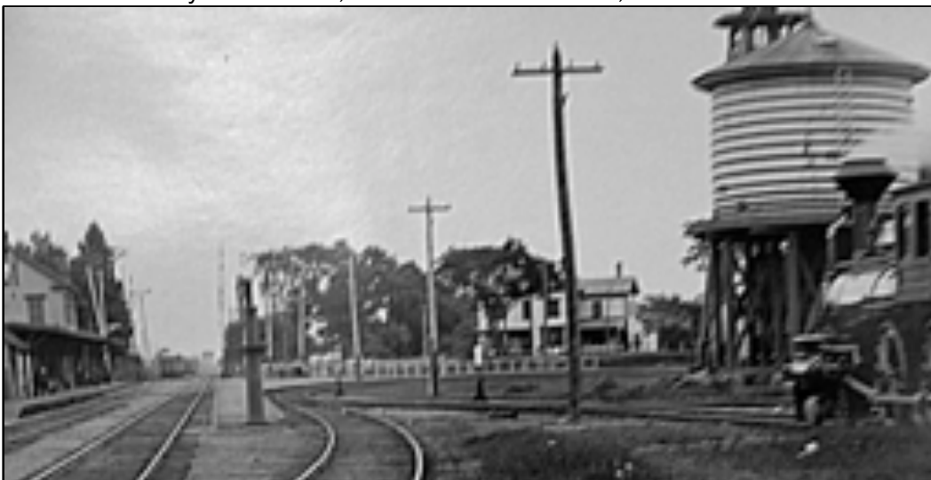
Hamilton began installing in 1930, water mains for fire purposes. First water main was on Railroad Avenue from Main Street to Willow Street. It had four hydrants. Pressure for the mains came from a water tower at the railway depot. Photo, Hamilton Historical Society
