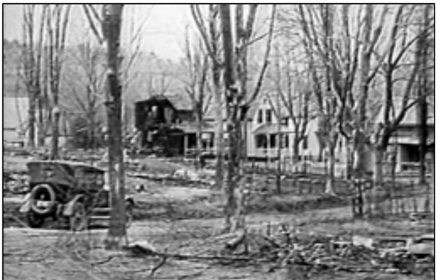
1927 Asbury Grove Fire destroyed more than 100 cottages. Photo, Hamilton Historical Society
