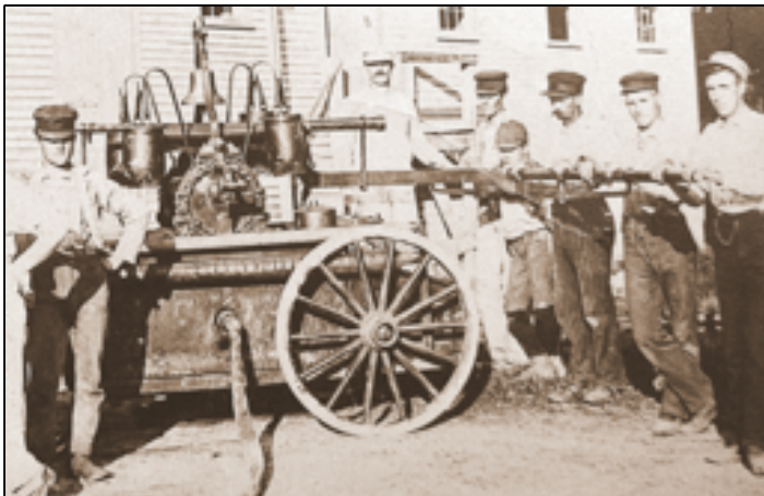
Working pump handles at 60 strokes per minute could pump 120 gpm. Fire fighters pulled the engine with ropes wound on reels below the tow bar, which also was used to steer the pumper. The rig was stopped by grabbing the pump handles. Photo, Hamilton Historical Society
