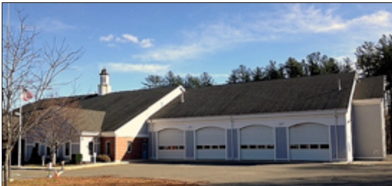
Public Safety Building , built in 2005, has police station, emergency response center and fire station. Garage has 4 bays; offices are on left and hose tower on right. Photo, J. Hauck, 2018
