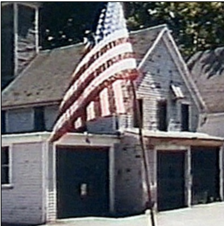
Willow Street engine house closed in 1957. Photo, Hamilton Historical Society
