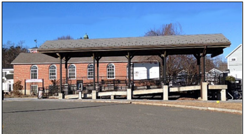
Elevated platform , at Hamilton-Wenham station. Brick building at back originally was a wooden freight house on east side of tracks. Photo, J. Hauck, 2019
