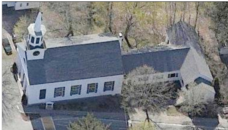
In 1953, the vestry ( right ) was raised and a kitchen and hall built underneath. A connection, built between the sanctuary and the vestry, provided office and classroom space. Photo Microsoft and Navteq
