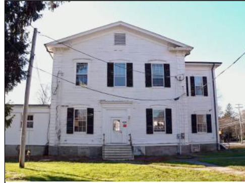
Side entrance removed in 2007. Photo J. Hauck, 2007
