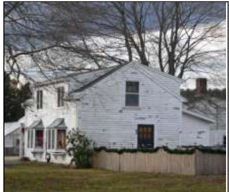
93 Main St., built 1870. Photo J. Hauck, 2012
