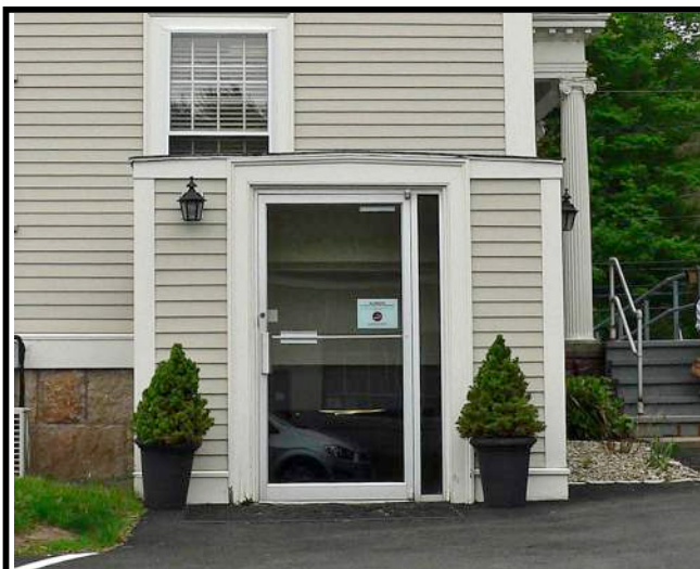
Fig. 40: Enclosed entrance to basement was rebuilt in 1979. Photo, J. Hauck, 2014.
