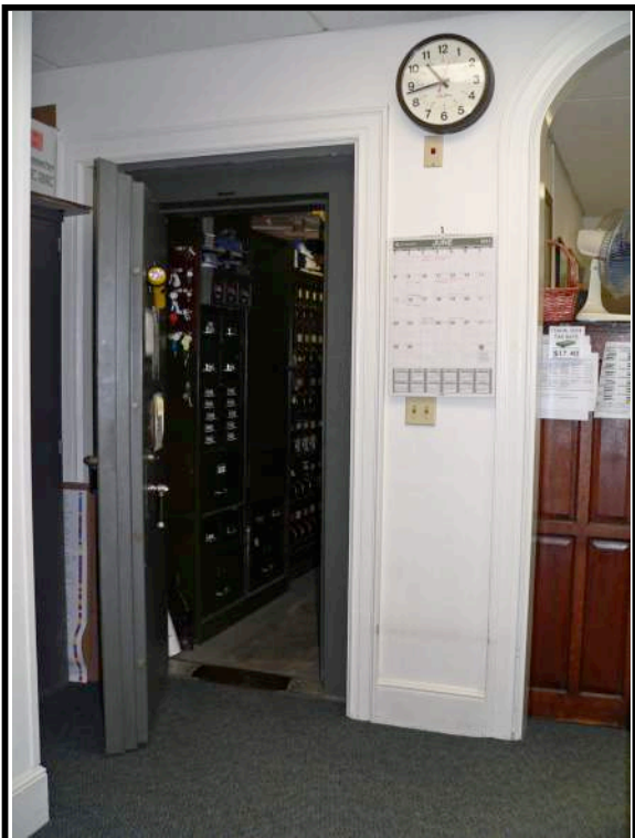
Fig. 56: Vault was built in town clerk's office in 1953. Photo, J. Hauck, 2014
