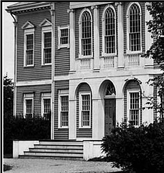
Fig. 7: Windows on each side of the front entrance doors are set in an arched niche. Photo, F. C. Norton, 1900
