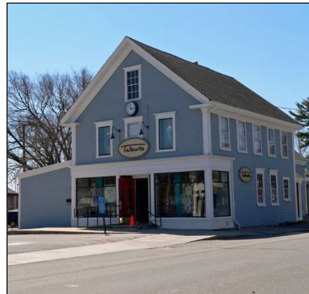
2014 - Talbot's store , other than sign change, remains the same as it did when it opened in 1993. Photo, J. Hauck, 2014
