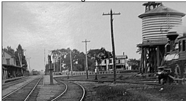
1900 - Water tank , on east side of railroad tracks, provided pressurized water to hydrants on Railroad Ave. Photo, courtesy Wenham Museum
