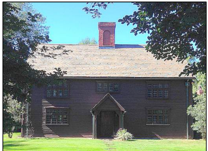
Old Tavern, 9 Farms Rd. was Hamilton's first post office. Samuel Story, Jr. was the first Postmaster, serving from 1803 to 1841. Photo, J. Hauck, 2015.
