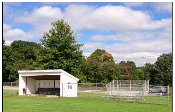
2016 bleacher stand built, followed in 2017 by dugouts. Photo, J. Hauck, 2018
