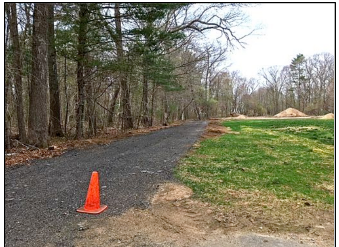
New road in construction. Photo, J. Hauck, 2018.
