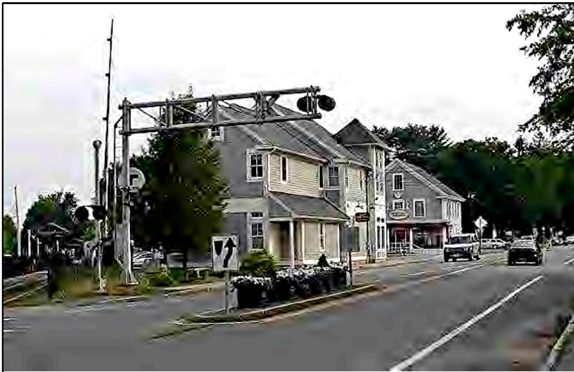
RR crossing , on Bay Rd., also has a gate on Walnut Rd. Photo, J. Hauck, 2016.
