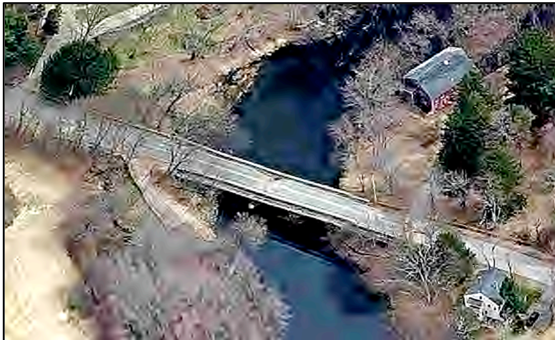
Highland Street Bridge , built in 1833 over Ipswich River, has field stone construction with triple arches. Photo, Bing Maps, 2015.
