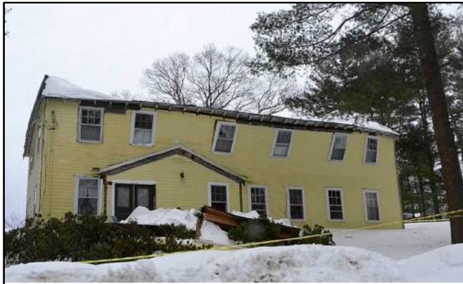
Fletcher Hall , former Swedish tabernacle, had major damage when snow-laden roof collapsed in March 2015. Building was later removed. Photo, AG Historical Society
