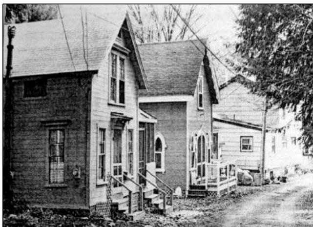
Stove pipes, ( far left ) were on sides of many cottages. Chimneys were not allowed. Photo, Salem Evening News,
