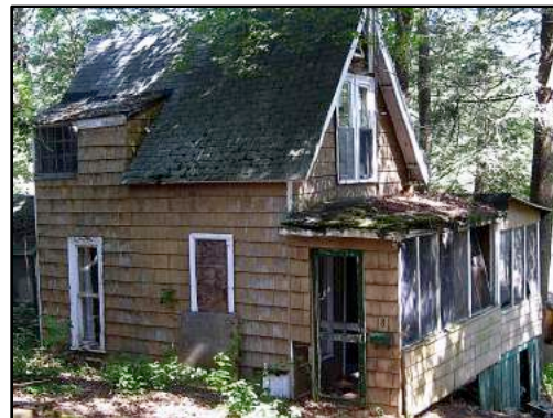
Platform , 8 Baker Ave., allowed cottage to be built on slope. Photo, J. Hauck, 2016
