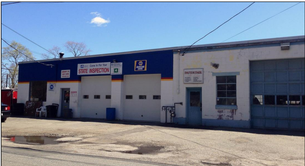
Patton Park Auto Body moved into the shop at the south end of Willow St., in 1981. Asbury Street Car Care , in 2014, moved into 2 bays and an office, on the Asbury Street end of the building.
