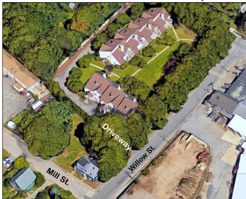
300 Willow St. , since 1986, is a residential condominium. There are 7, 2-story units, each with about 3,600 sq. ft. of living space, and an attached garage. Photo, Bing Maps, 2015.
