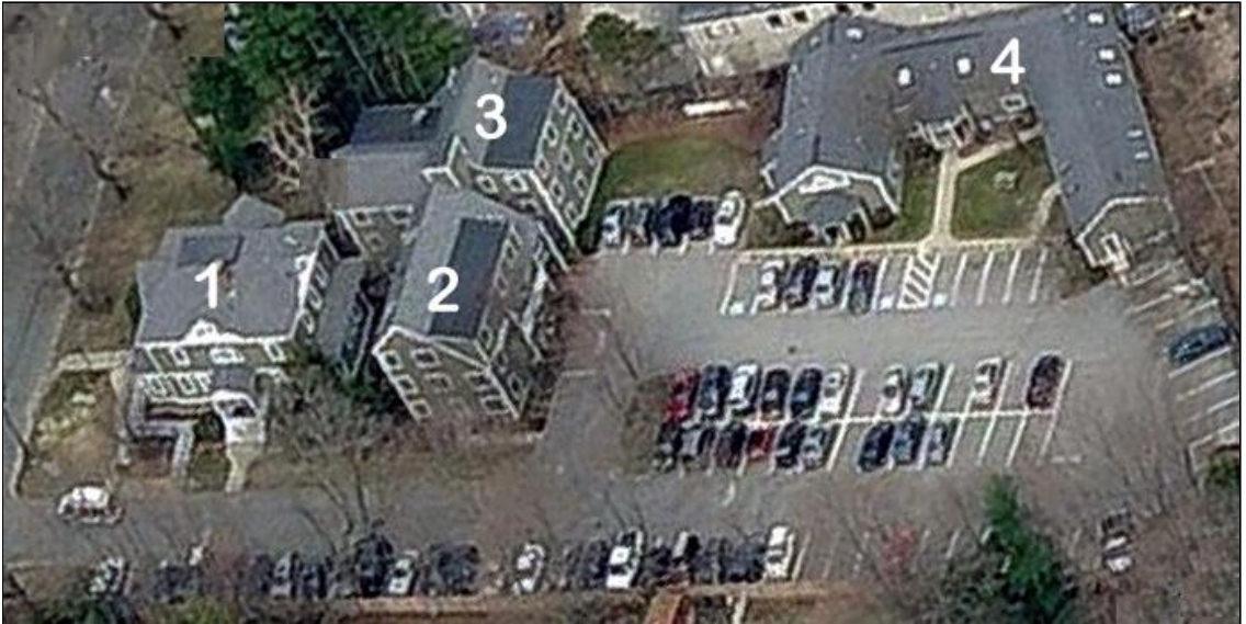
203/205 Willow St. became the Willowdale Center office park in 1970. There are 4 units and a large parking area. Photo, Bing Maps, 2012
