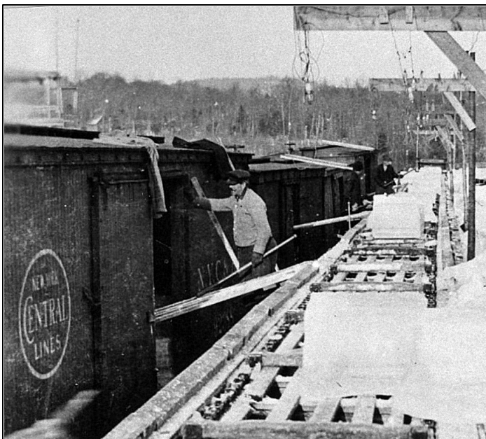
Ice blocks were loaded in insulated railcars, on siding near icehouses. 34-ft. cars generally could hold \sqrt{80} tons of ice.
