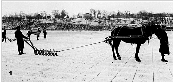
1 Groove cutter , increased the groove depths to about 2/3rds the ice thickness. Photo various
