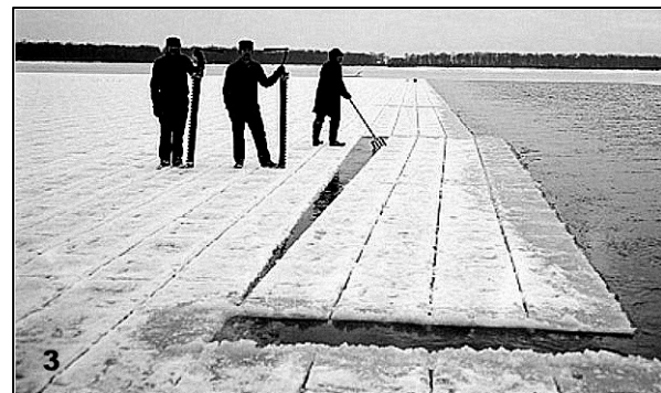
3 Floats sawed from field and guided into main channel separation into strips. Oldhouse web
