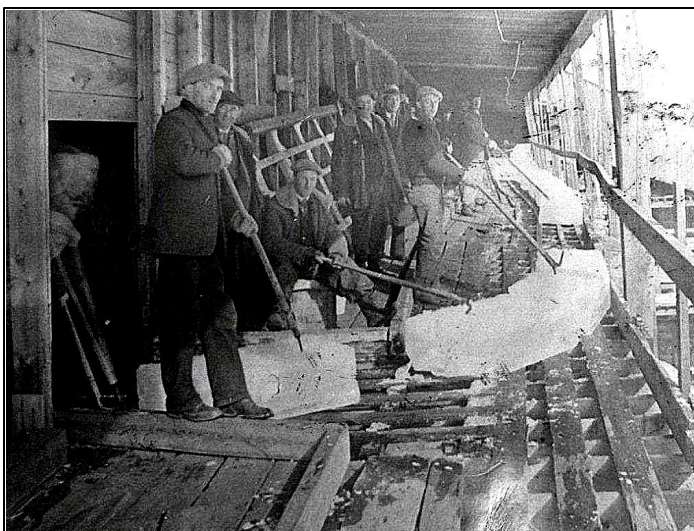
Workers moved ice blocks along loading platform to openings in icehouse. Photo, Hamilton Historical Society
