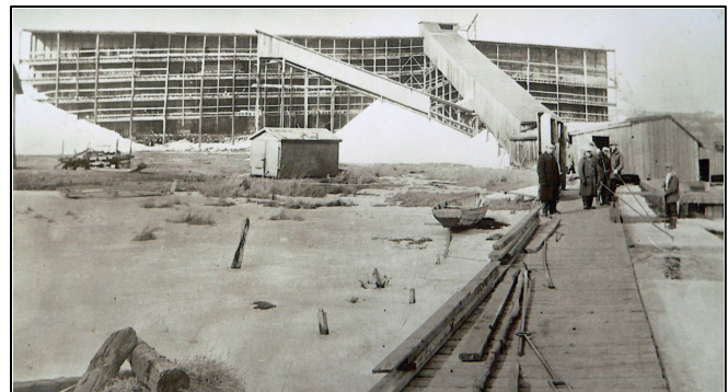
C. W. Mears icehouse , built in 1900, was on the Essex Shore of Chebacco Lake. Located at the end of Patriot's Landing, it could hold more than 40,000 tons of ice.
