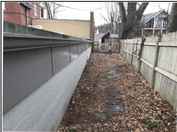
No windows in walls of addition's back section. Photo, JHauck, 2022
