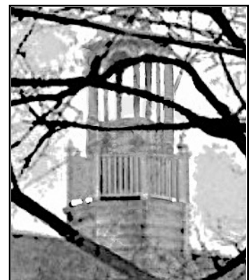
Wood railing on cupola deck was removed in 1993.
