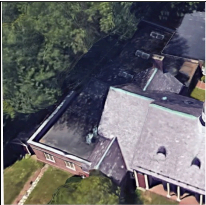
Three skylights on back of addition roof Photo, Google, 2021
