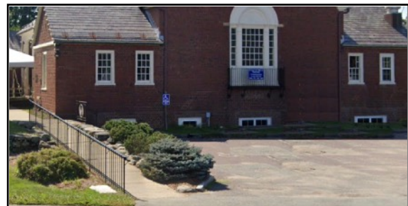
Handicapped ramp and easily opened door locks and lights were installed by walkways around the building, in 1986.
